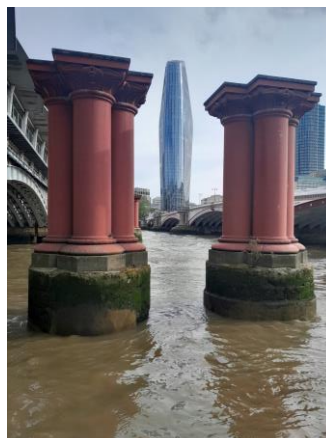
Remains of the old Blackfriars Bridge
